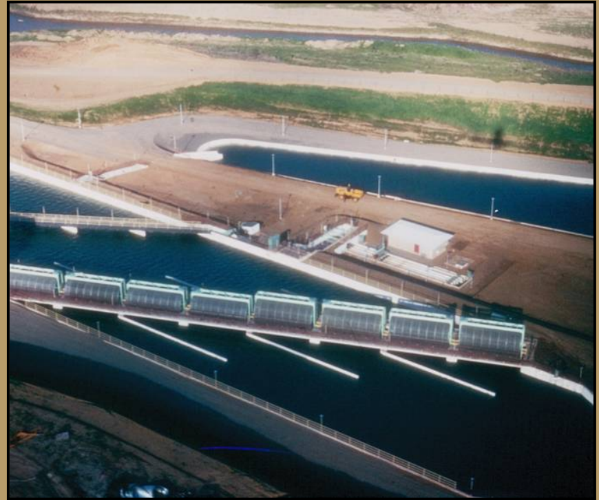
Fish Protection Facilities, PNR
