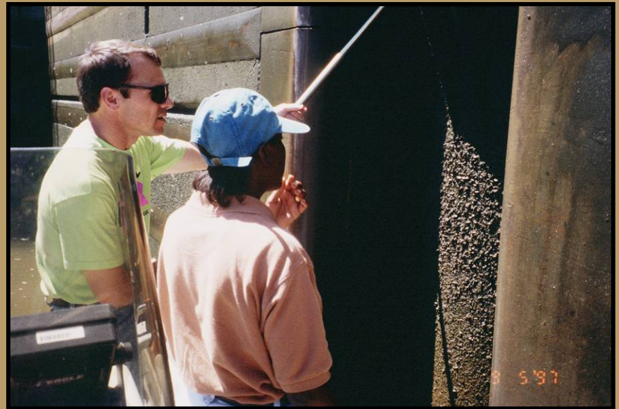
Kerr Lock and Dam (COE), Tulsa OK
